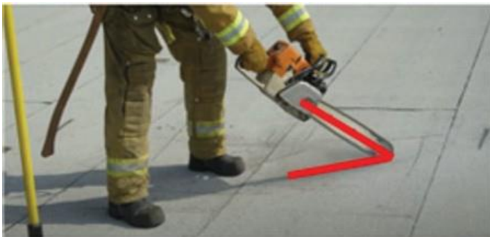
Avoid kickback by using a shallow angle to begin cuts
